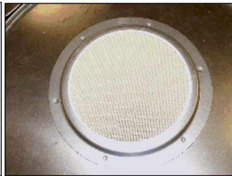
Bottom view of flame arrestor.
